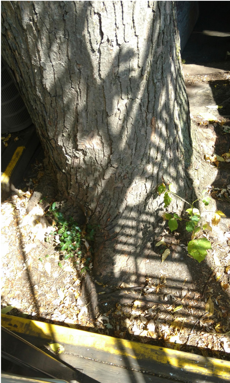
IMAGE 4 – Exposed Roots, Damaged (TREE 2)
