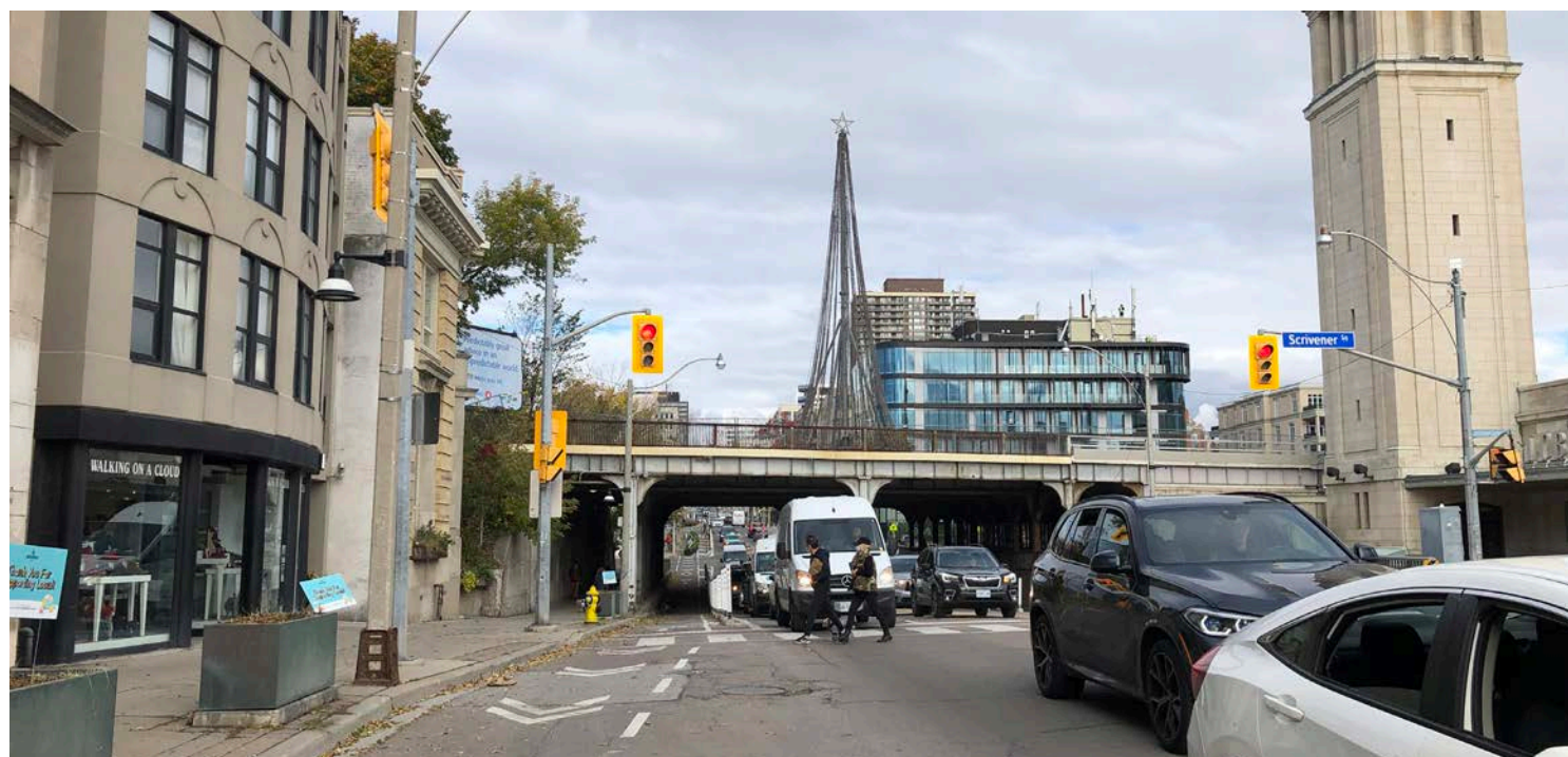
Figure 17. At the south of the Block, the view toward the Subject Site is obscured by the CP Rail bridge
