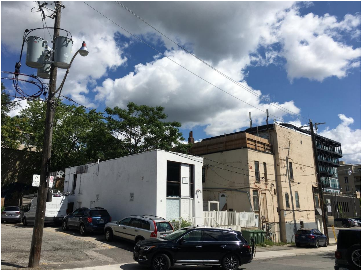
Figure D-3 View from South of Birch Ave of the hydro poles located at sample locations A1 and A5
