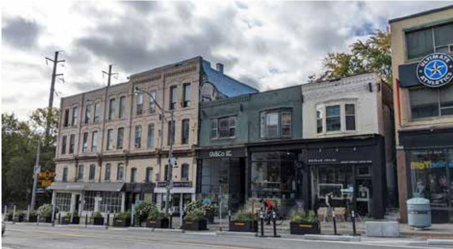
View of Buildings A and B from the east side of Yonge Street (ERA, 2021).
