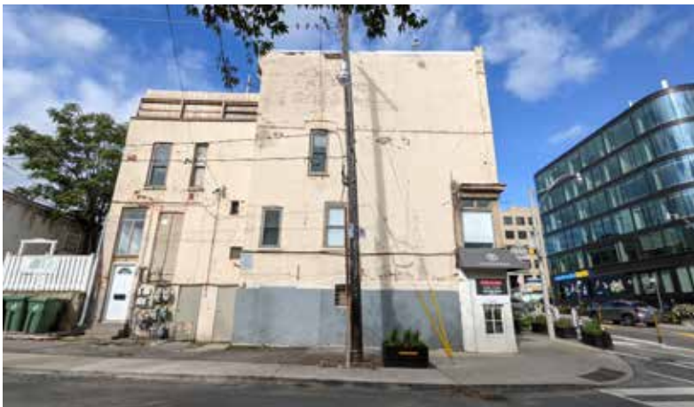
South elevation of Building A (ERA, 2021).
