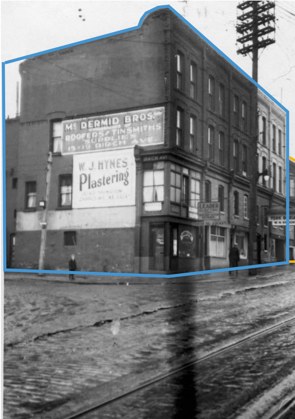
1935, view looking northwest to the corner of Yonge Street and Birch Avenue. The new first storey of Building A (outlined in blue) has been retrofitted with shop windows (City of Toronto Archives, annotated by ERA).
