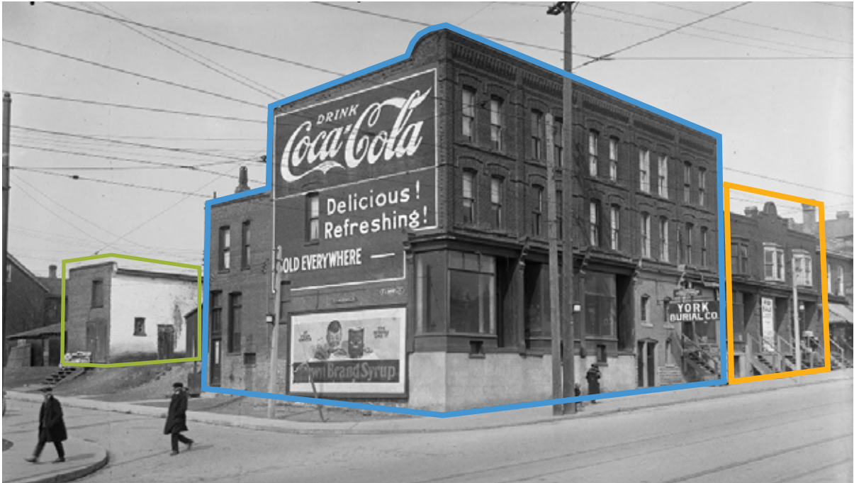
1920, view of northwest corner of Yonge Street and Birch Avenue that shows Buildings A (outlined in blue), B (outlined in yellow) and C (outlined in green). The exposed basement of Building A is enclosed with only one staircase entrance at the north bay, staircases have been installed to access the shops in Building B (City of Toronto Archives, annotated by ERA).
