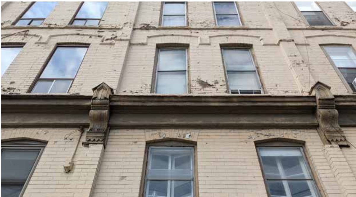
Remnant wood cornice on Building A marks the top of the original retail bays, now located at the top of the second storey (ERA, 2021).
