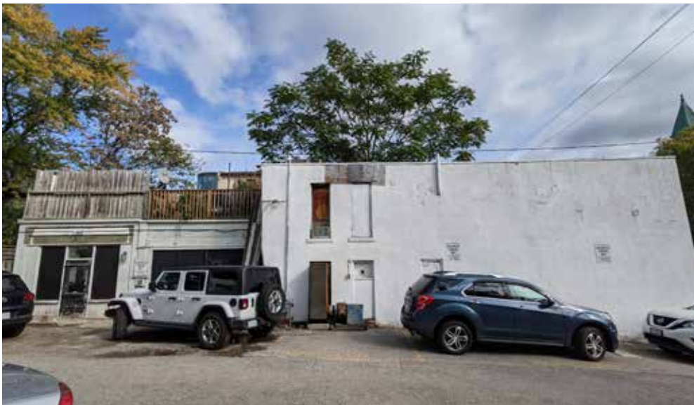
West elevation of Building C (ERA, 2021).
