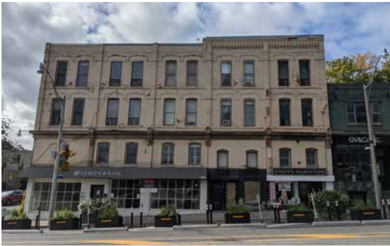
East elevation of Building A (ERA, 2021).
