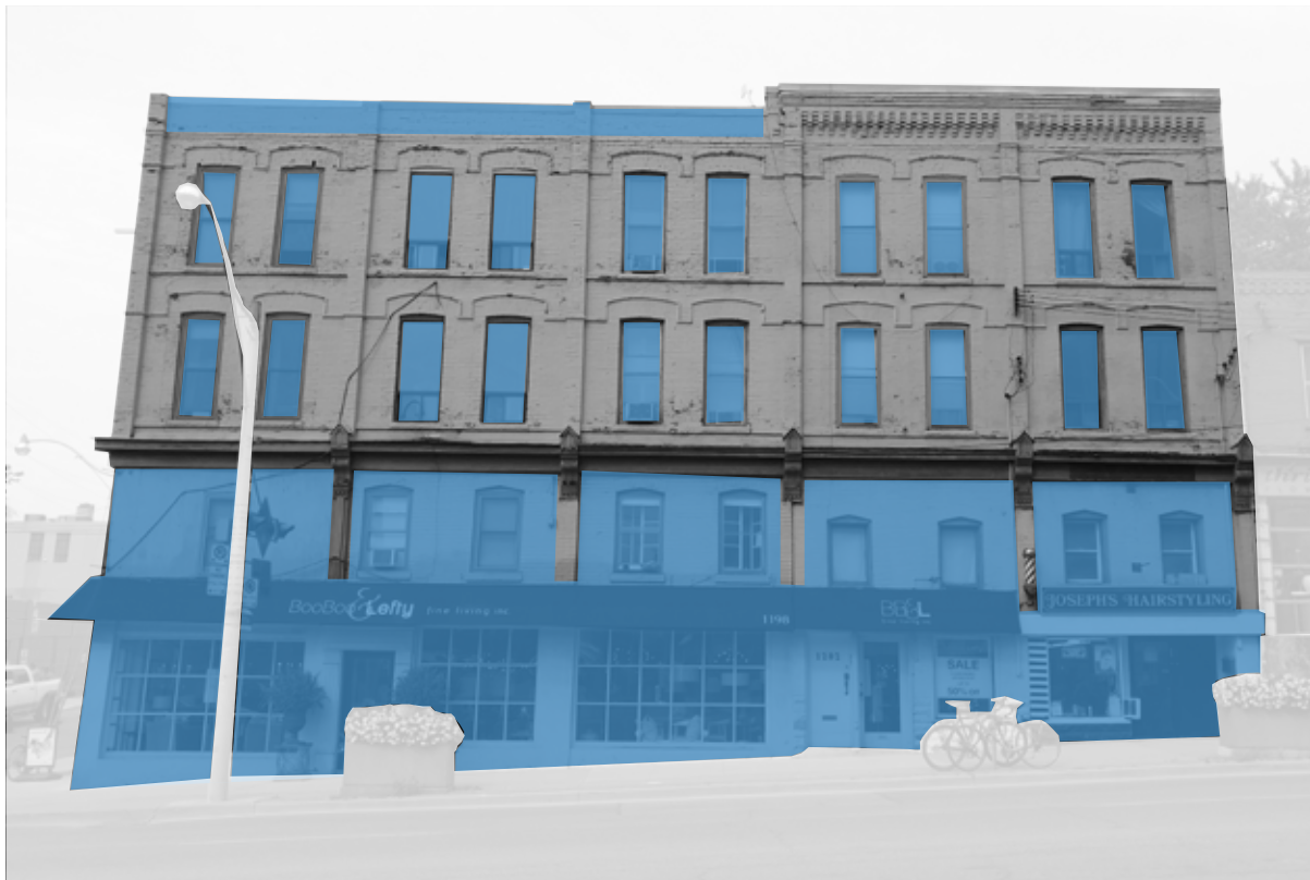
Building A, east elevation. All images are marked in blue where alterations have occurred (ERA 2017).
