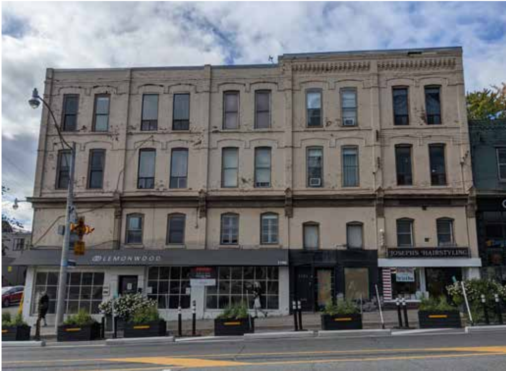
East (principal) elevation of Building A (ERA, 2021).
