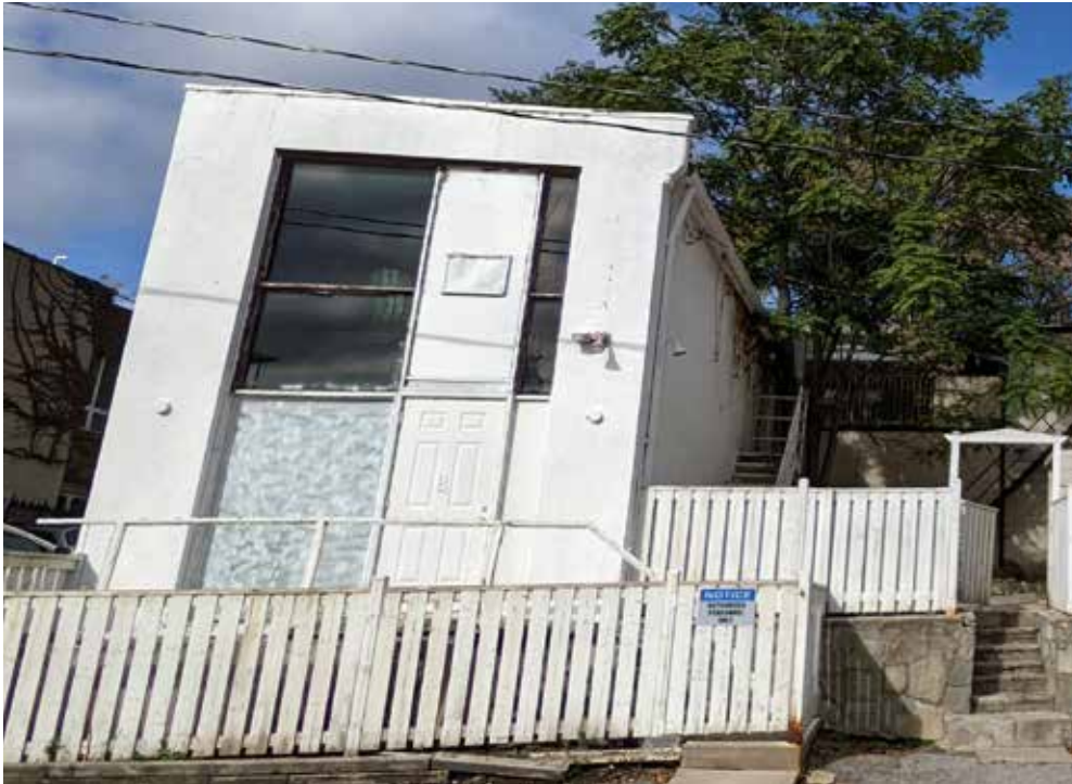
South elevation of Building C (ERA, 2021).
