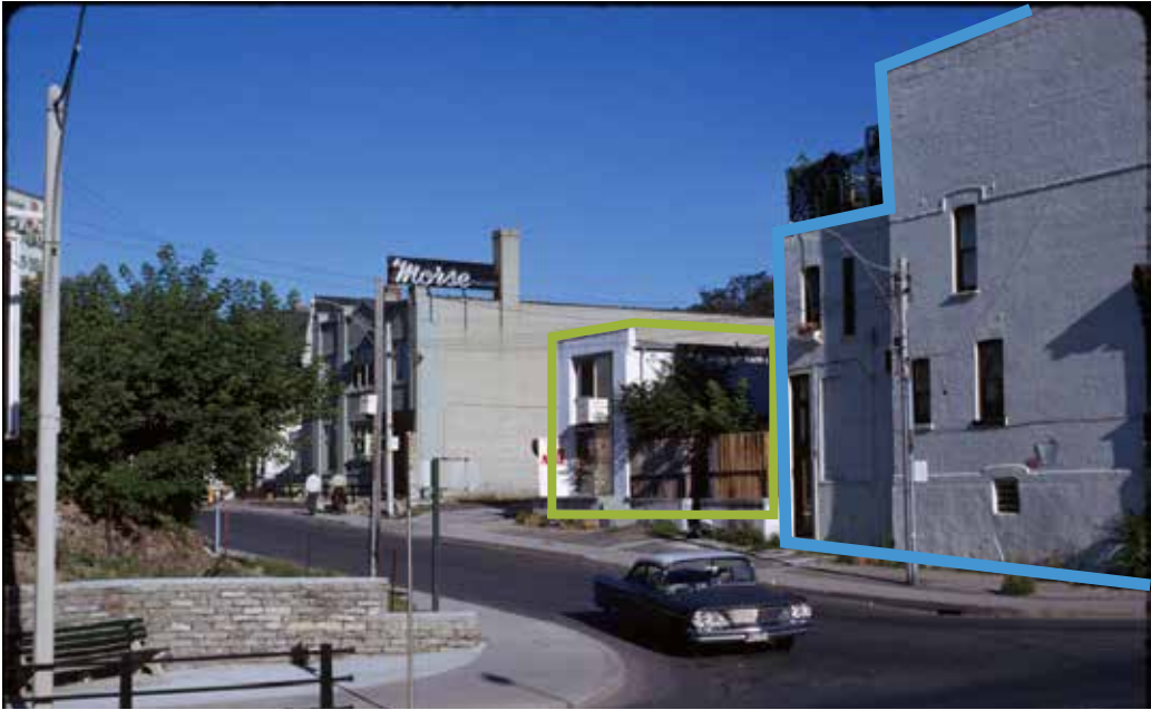
1973, A portion of the south elevation of Buildings A (outlined in blue) and C (outlined in green) (City of Toronto Archives, annotated by ERA).
