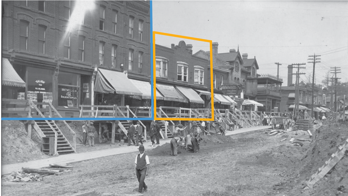
1914-1916, view looking west from the east side of Yonge Street, Building B (outlined in yellow) and part of Building A (outlined in blue) during the regrading of Yonge Street (City of Toronto Archives, annotated by ERA).
