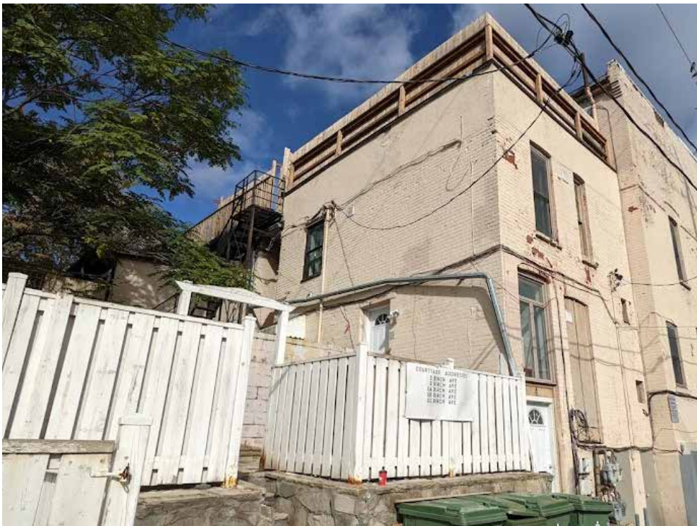
West (rear) elevation of Building A (ERA, 2021).
