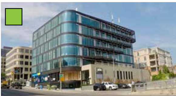
6-storey post-modernist office building constructed c. 1986, and reclad in 2016 for office and retail use.
