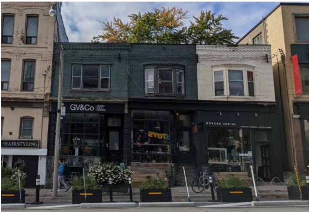
East (principal) elevation of Building B (ERA, 2021).
