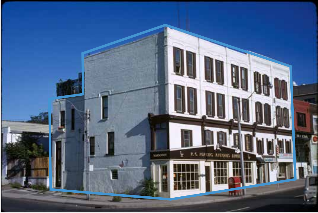
1973, view from the southwest toward to the northeast corner. The photo shows south and east elevation of Building A (outlined in blue). The building had been painted white with dark accents, shutters were installed on the east elevation windows (City of Toronto Archives, annotated by ERA).
