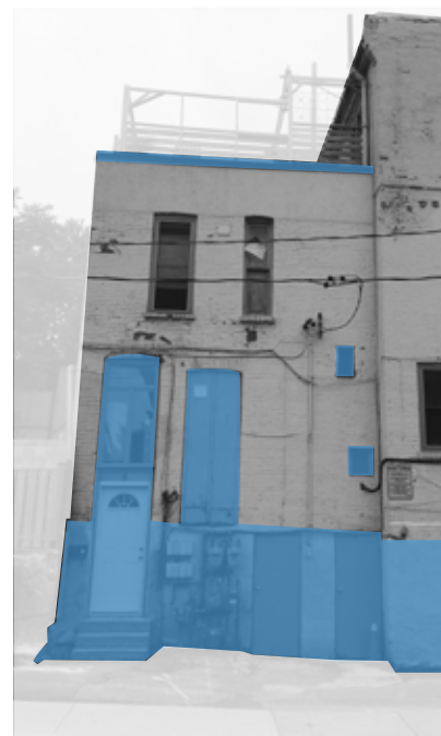
Building A, south elevation (ERA 2017).
