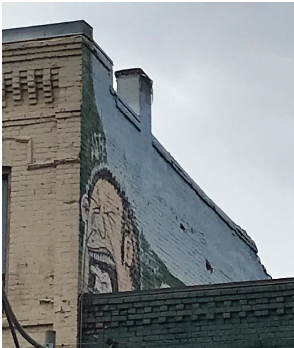
Metal parapet flashing in fair condition (ERA, 2021).
