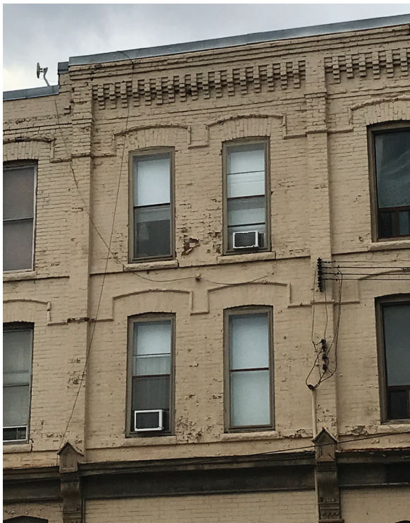
Photos of east elevation of Building A shows cracking, open and deteriorated mortar joints, and peeling paint. Deteriorated and damaged brickwork includes spalled, fractured, eroded, missing masonry units, obsolete fasteners and holes in the bricks (ERA, 2021).
