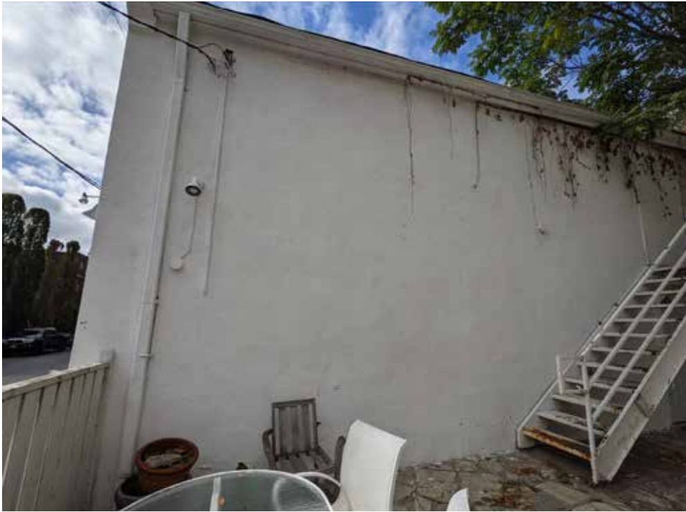
East elevation of Building C (ERA, 2021).
