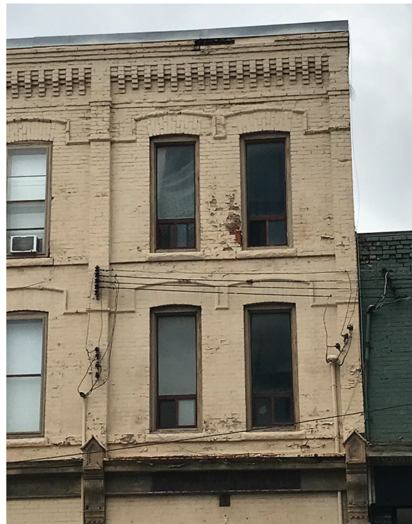
Photos of east elevation of Building A shows cracking, open and deteriorated mortar joints, and peeling paint. Deteriorated and damaged brickwork includes spalled, fractured, eroded, missing masonry units, obsolete fasteners and holes in the bricks (ERA, 2021).
