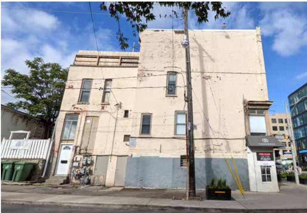
South elevation of Building A (ERA, 2021).
