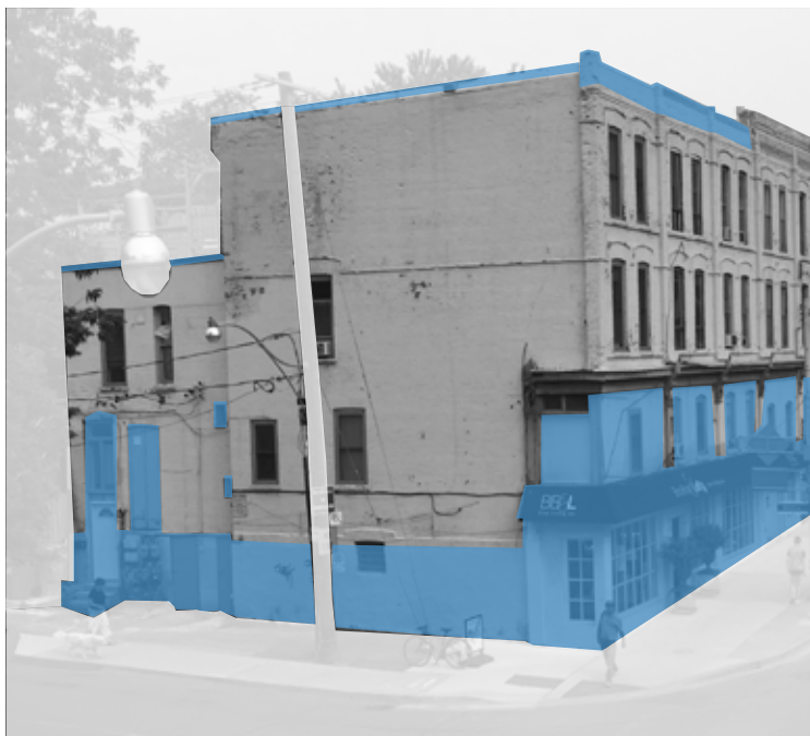
Building A, south elevation (ERA 2017).
