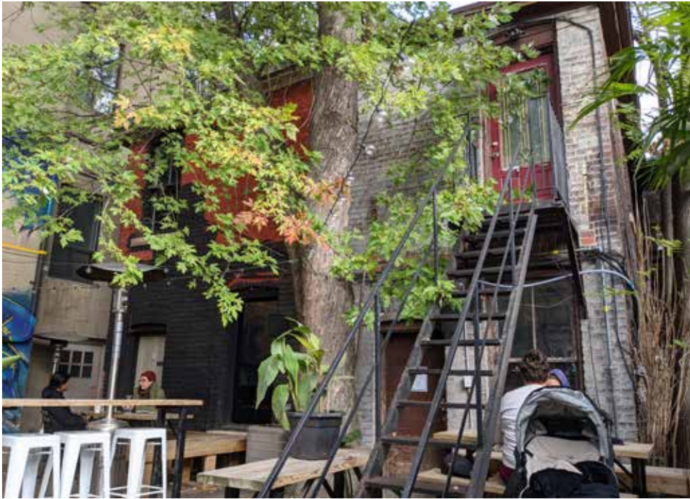
West (rear) elevation of Building B (ERA, 2021).
