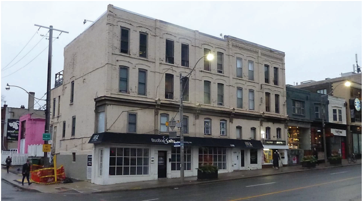
Photo #1: General view of east elevation of 1196 – 1210 Yonge Street, Toronto
