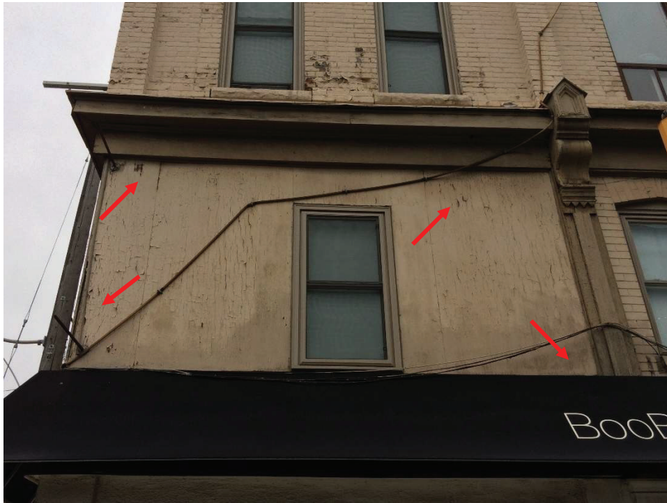
Photo #9: General view of plywood covering at Unit 1196, 2 ND Floor. Plywood appeared to be undergoing deterioration.
