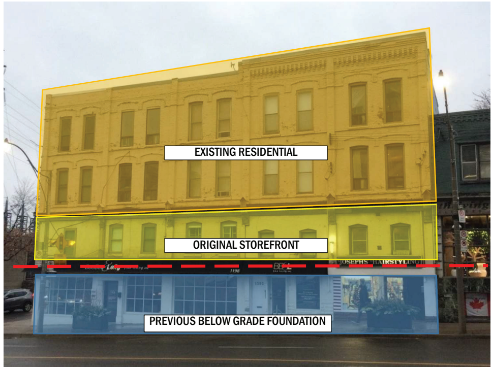
Photo #5: View of various historical modifications due to Yonge Street re-grading at Building 'A'. The approximate line of original grading at time of construction is shown in red. The previous basement and current ground floor storefront is shown in blue. The previous storefront and current 2 ND Floor shown is shown in yellow. The existing upper residential floors, shown in orange and appears to be mostly unchanged from the original construction.
