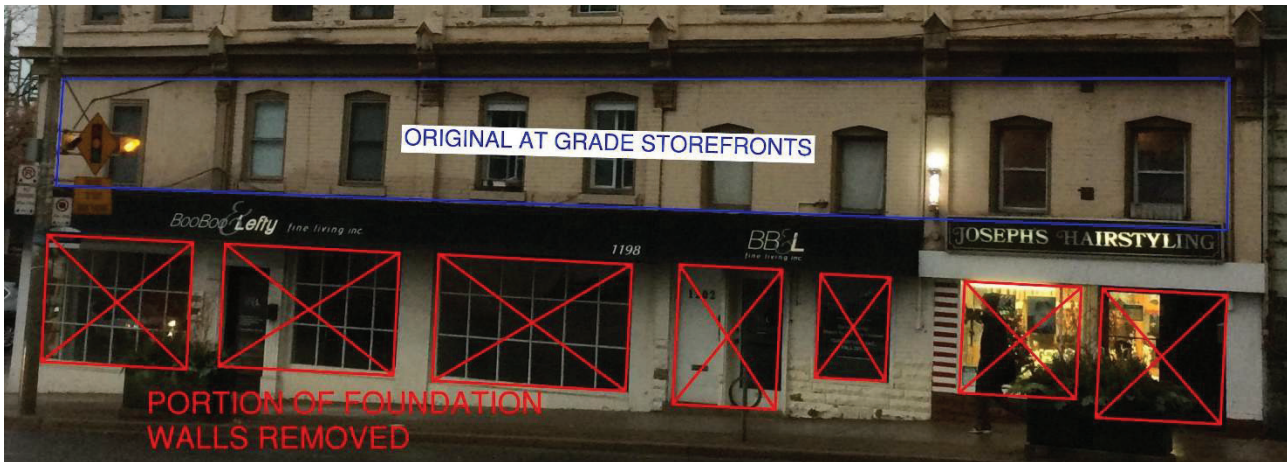
Photo #6: Building elevation outlining large sections of original basement foundation walls previously removed.
